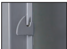
Main door latch hooks welded to frame
